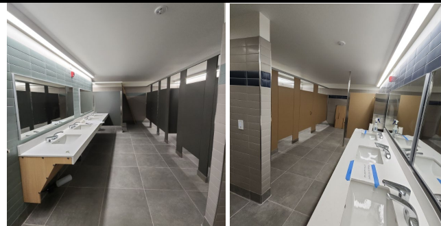
Interior Restroom - Building 800
