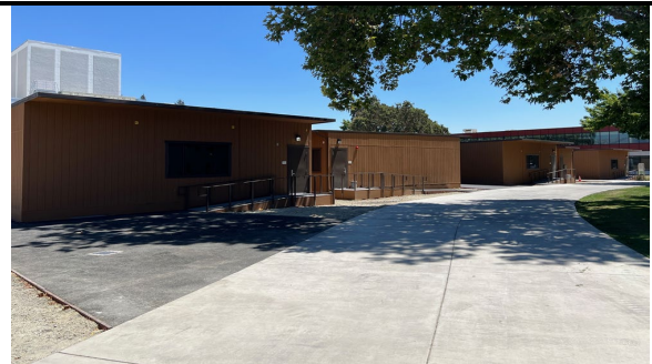
Modular Classroom Installation
