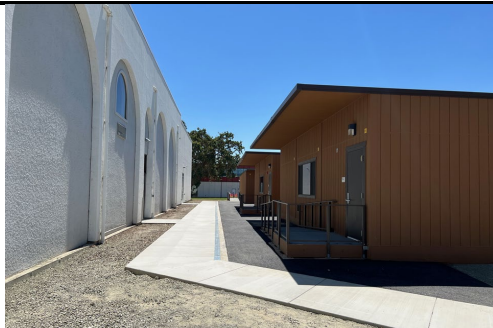
Modular Classroom Installation
