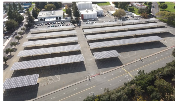
New Solar Canopy Installation
