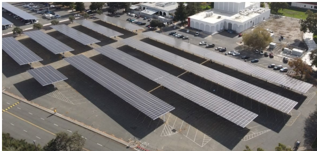
New Solar Canopy Installation
