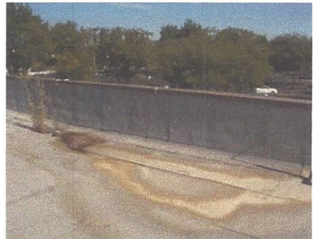
Evidence of water ponding
