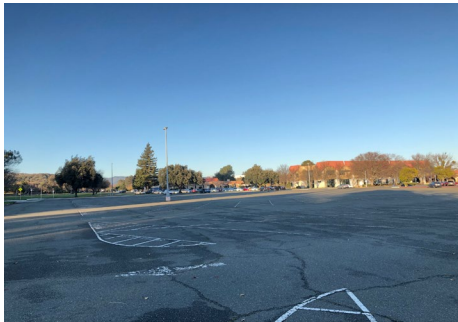
Existing Parking Lot #01
