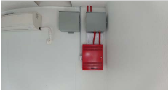
Completed Fire Alarm System Installation
