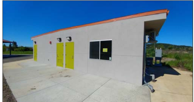
Modular Restroom Building and Surrounding Hardscape
