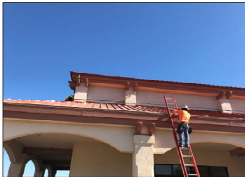
Decorative Wood Corbels to be Removed Due to Dryrot Issues
