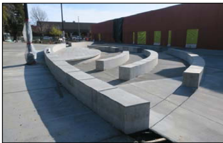
Stage & Seat Walls at Entry Courtyard
