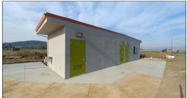
Modular Restroom Building and Surrounding Hardscape
