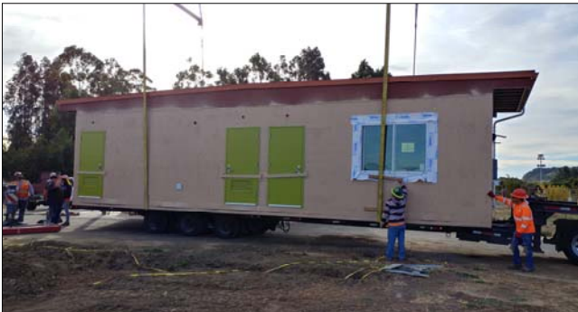
Crane Hoist of Modular Building onto Concrete Foundation
