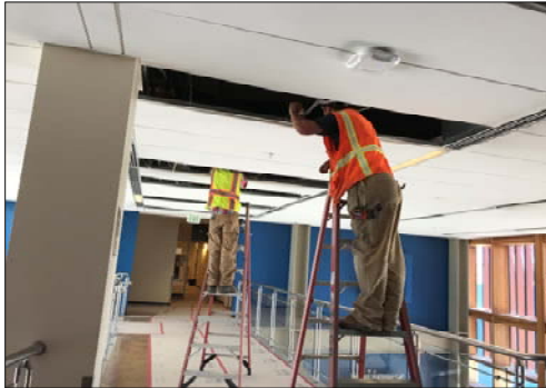
Installation of New Ductwork
