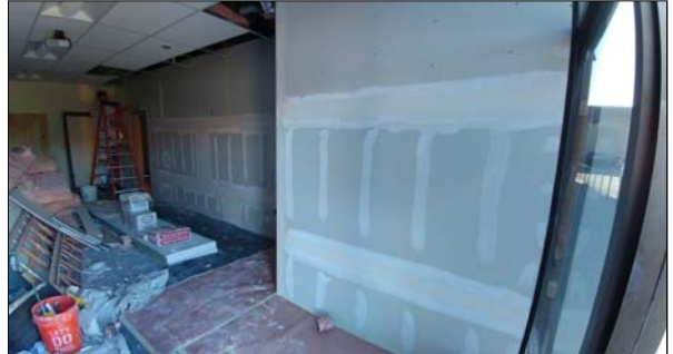
Taping and Finishing of Sheet Rock
