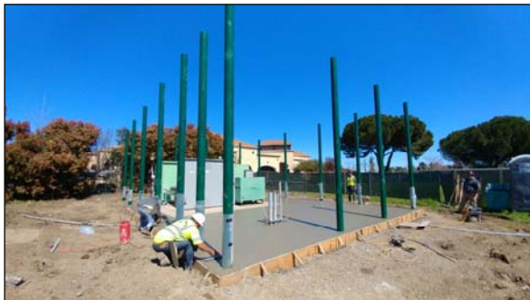
Finishing Concrete Pad for New Generator
