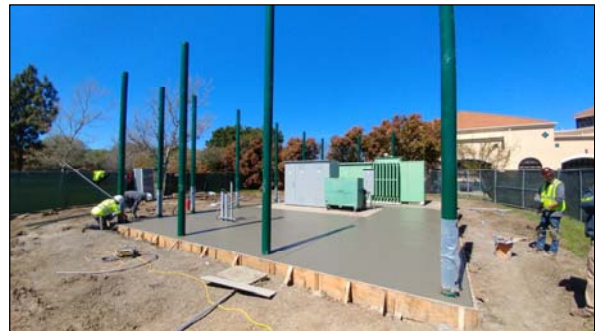
Concrete Pad & Fence Posts for New Generator
