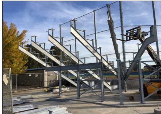
Erection of Bleacher Structural Steel
