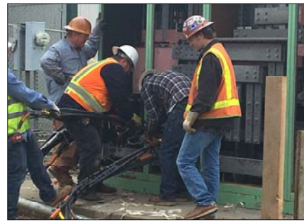
Connecting Power Feeds at Substation #1
