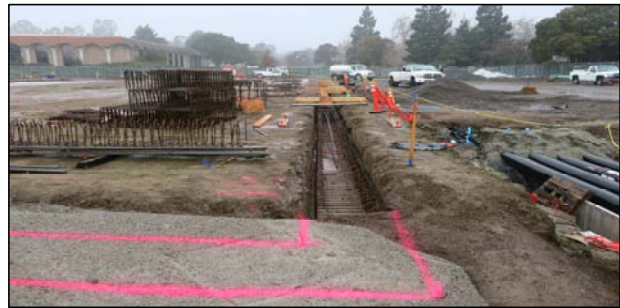
Installation of Reinforcing in Foundations
