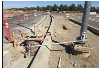
Relocating Light Pole
