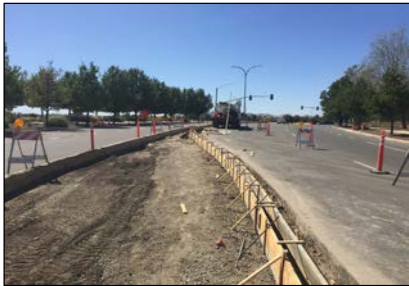
New Work in the Street
