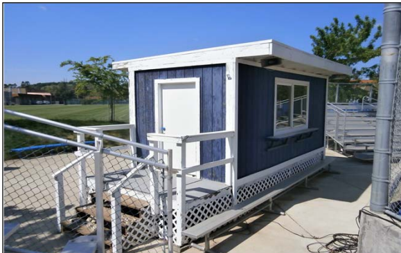
Old Press Box to be Removed and Replaced
