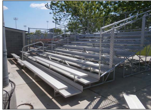
Old Bleachers to be Removed and Replaced
