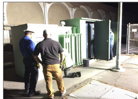
Substation #2 Being Evaluated
