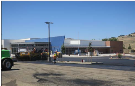
Site Paving in Progress
