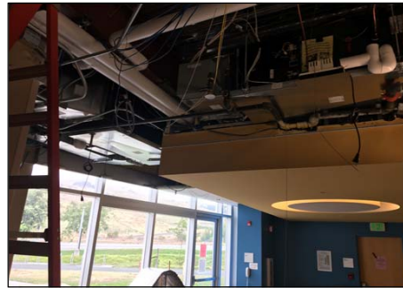
Work on System in Ceiling
