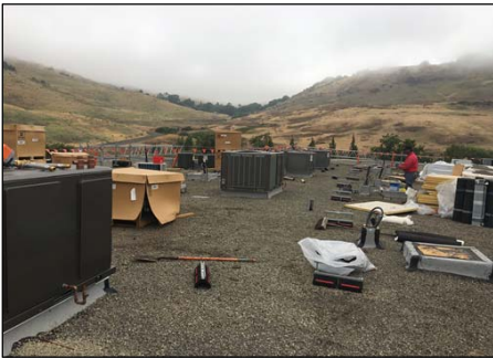
New HVAC Units on Roof
