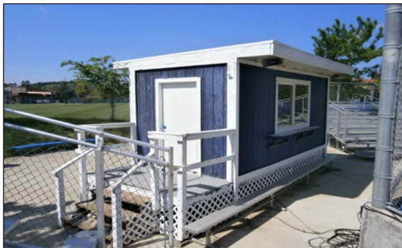
Old Press Box to be Removed and Replaced
