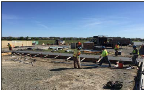
Exterior Flatwork In Progress
