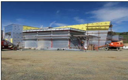
Building Entrance, Exterior Insulation at Walls
