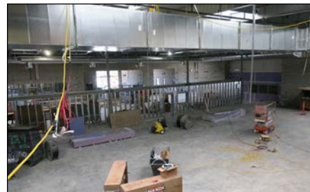
Ductwork and Framing at Instructional Bays
