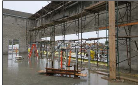
CMU Wall Construction
