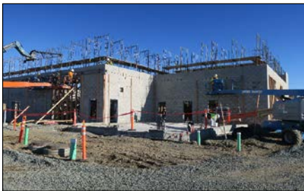
Installation of Ledger Beams
